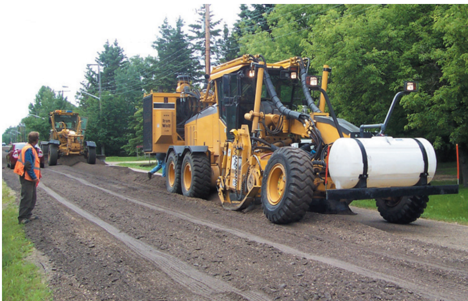
IronWolf started in the 1990s working with local contractors in Prudhoe Bay, Alaska trying to improve the arduous task of ripping the Alaskan permafrost. Beller's hard work and persistence led to the development of the IronWolf Crusher which successfully created a new and accepted process to make roadbeds.
